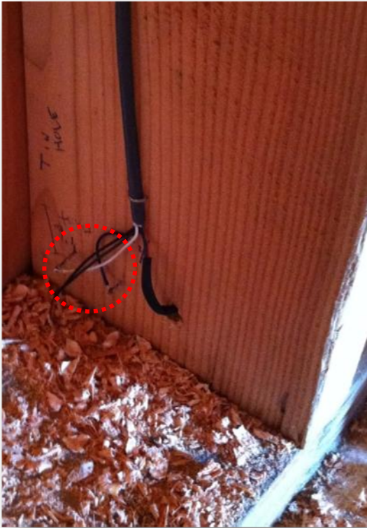
Figure 9. Resistance-based brass pins nailed to the wood studs were used for wood moisture content measurements. The black wires are attached to the temperature sensor.
