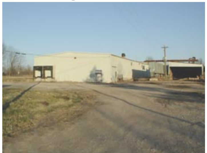
GO Inc.'s sustainable living demo project in an old flakeboard plant in Evanston, IL. We'll have the full story.
