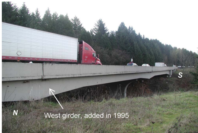
Fig. 2. Photo of the tested bridge
