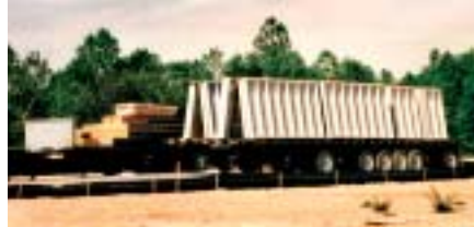
Photograph 10 Pre-cast basement walls
