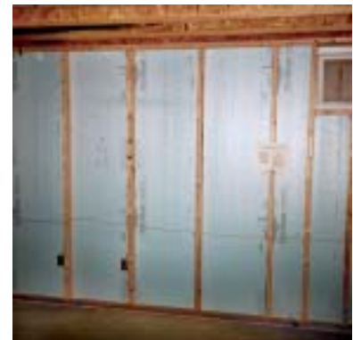
Photograph 9 Unfaced extruded polystyrene against basement wall
