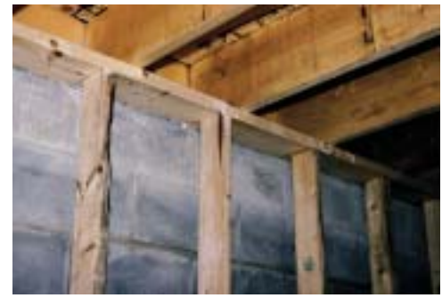
Photograph 1 Interior stud framing located at basement perimeter
