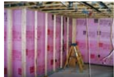
Photograph 8 Unfaced extruded polystyrene against basement wall
