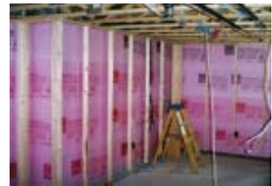
Photograph 8 Unfaced extruded polystyrene against basement wall
