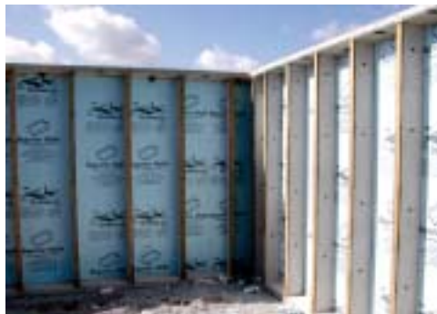
Photograph 11 Pre-cast basement walls with XPS foam insulation
