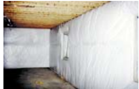
Photograph 3 Blanket insulation with impermeable vinyl interior surface
