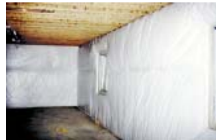
Photograph 3 Blanket insulation with impermeable vinyl interior surface
