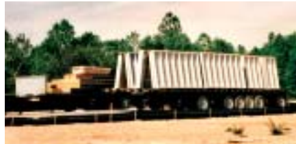
Photograph 10 Pre-cast basement walls
