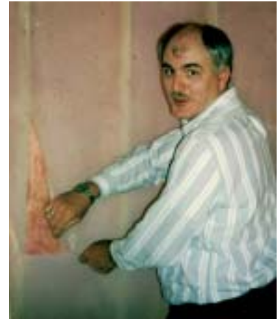
Photograph 2 Interior basement stud framing insulated with fiberglass batts and covered with a polyethylene vapor barrier
