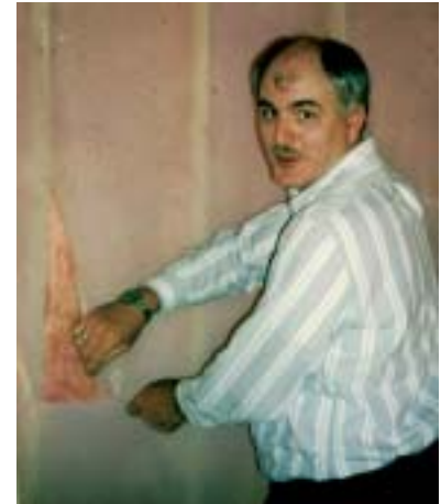
Photograph 2 Interior basement stud framing insulated with fiberglass batts and covered with a polyethylene vapor barrier
